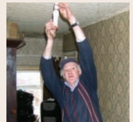
Installer Tim Enright fitting a low energy light bulb.
